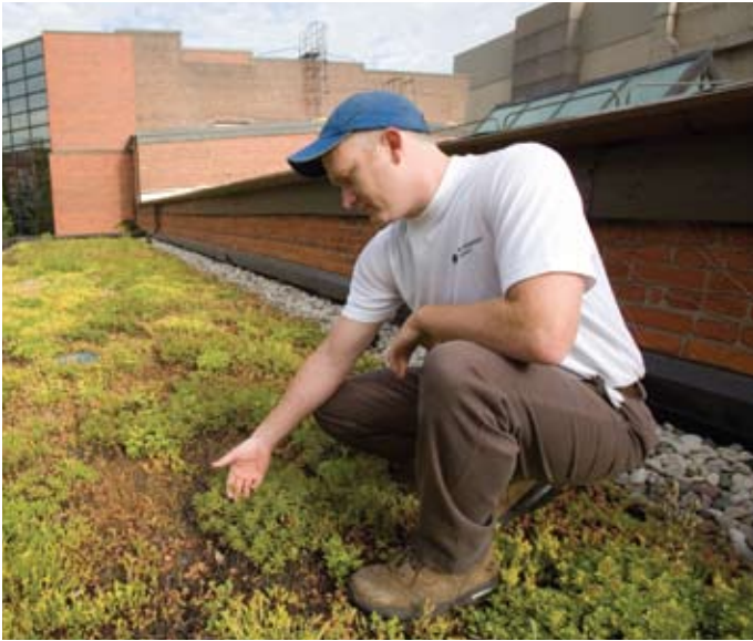
The first “living” roof in Louisville reduces our heating and cooling demands and decreases storm water runoff.
